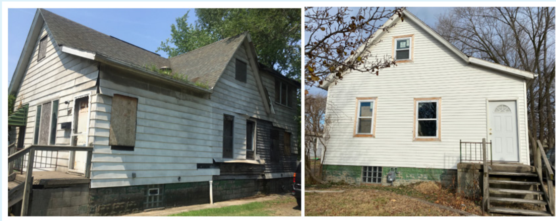
Before and After, renovated under a NAP Abatement Agreement – Wheelock, District 6.
