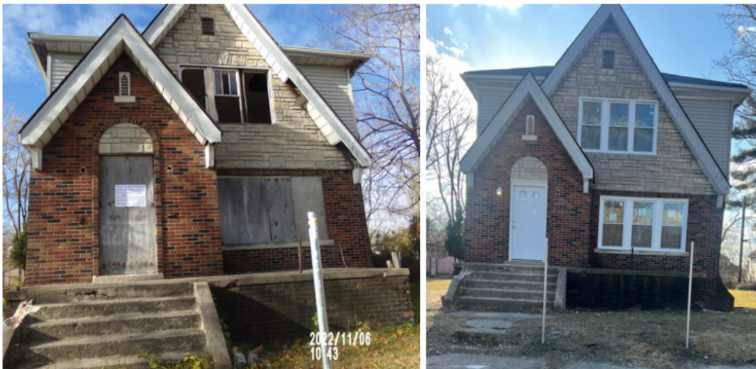
Before and After, renovated under a NAP Abatement Agreement – Gallagher, District 3.
