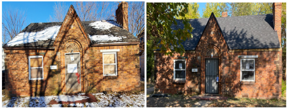
Before and After, renovated under a NAP Abatement Agreement – Marseilles, District 4.
